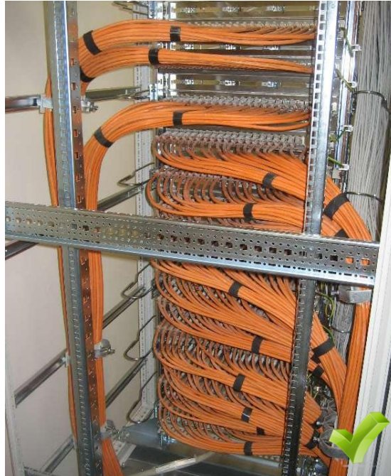
Figure 5: How to install and feed cabling from the side within an IT cabinet
