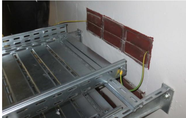
Figure 19: Interruption of metal cable management systems at fire wall
